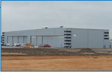
The exterior of the new paint facility was complete at the end of 2011 and is on schedule to open this spring.
