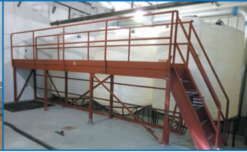
February 13, 2012 - Waste treatment room. The paint stripping waste is treated through a system of evaporators to minimize the amount of hazardous waste.
